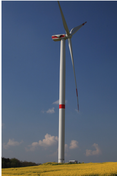
Fig. 2: Prototype of the W2E-120/3fc (3 MW wind turbine) erected in Kankel, Mecklenburg-Western Pomerania, September 2013
